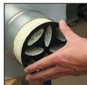
Druk de demper in de opening.
